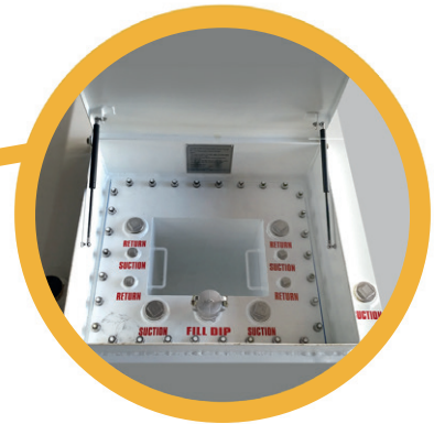
Tank Manway Recessed Spill Box Area
